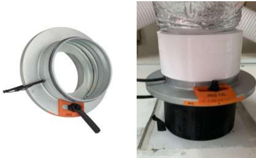
Fig. 2. Iris damper installed on top of square diffuser
