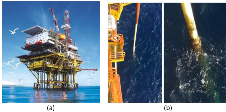
Fig. 1. Oil & Gas offshore (a) Host platform (b) Cylinder riser
