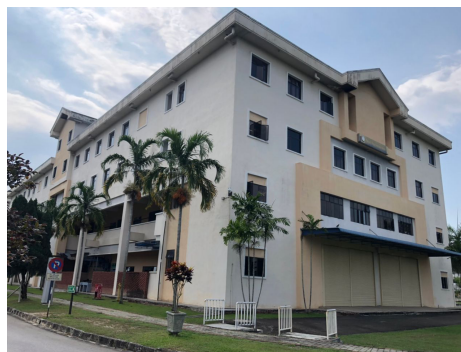
Fig. 1. FKM classrooms building
