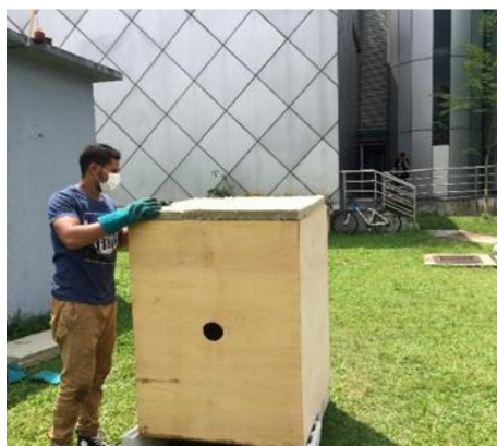
Fig. 2. Wooden Room Applying One Layer (50 mm) of Rockwool insulation
