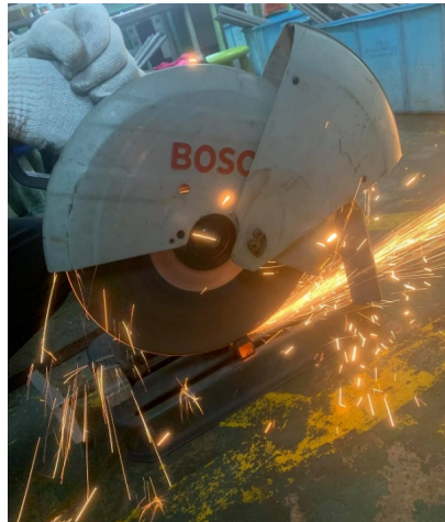
Fig. 9. Process of cutting the steel hollow bar
