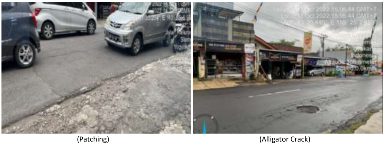
Fig. 6. Patching and alligator crack distress type
