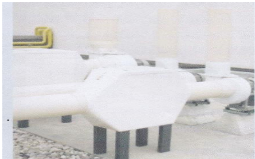
Fig. 1. Carbon Filtration System [6]
