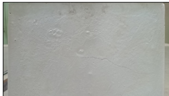
Figure 6: Crack on Exposed Face (900g Gypsum and 100g Kaolin clay of 9.5 mm).
