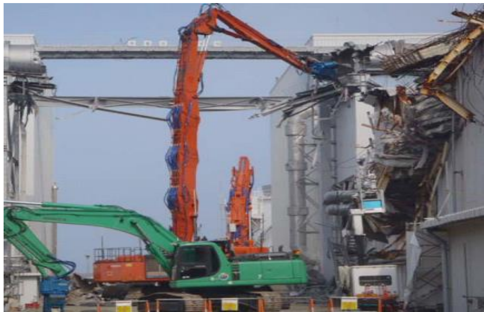
Fig. 4. Unmanned excavators at nuclear disaster area
