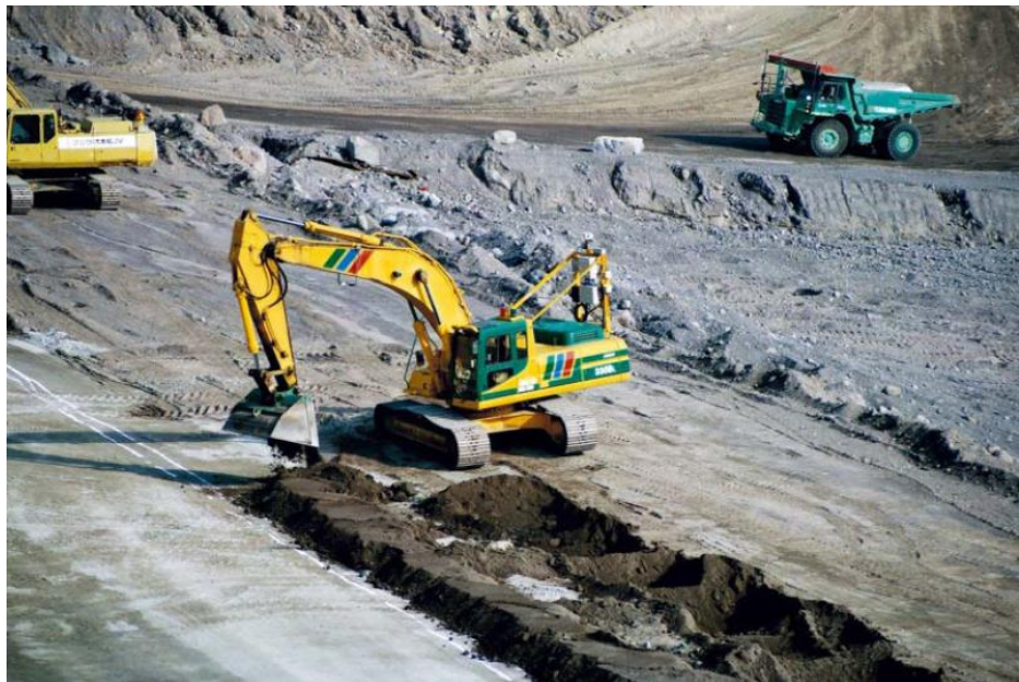
Fig. 3. Unmanned excavators in Sabo works
